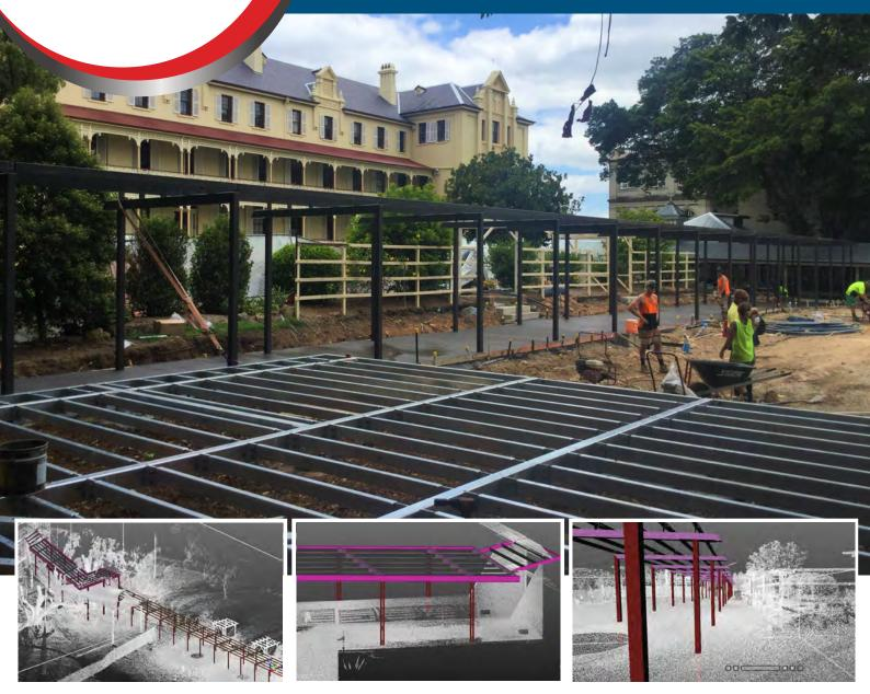
Using our 3D Scanning Technology and Robotic Total Station for site measurement, we were able to overcome the challenges of this project, which included uneven ground level and footings designed at varying heights. The accuracy of this technology enabled a seamless flow from measurement through to fabrication & installation, allowing us to complete the job within time-frame with no rectification works.
